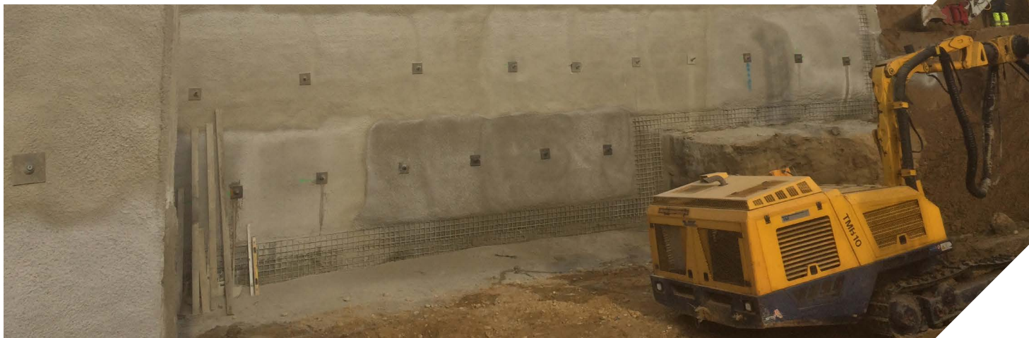
Soil nail with hollow bar
